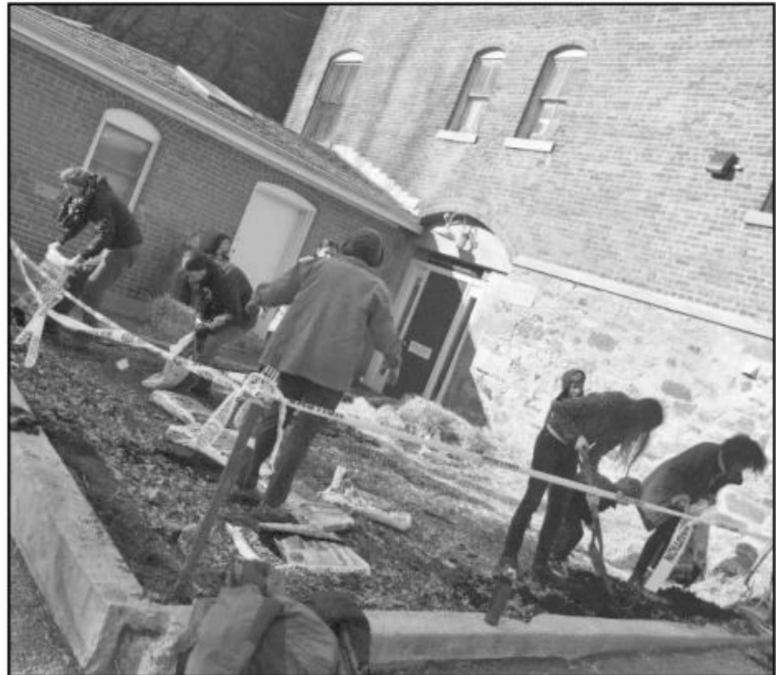
Volunteers dig out space at the Studio Around the Corner for the new community garden.
